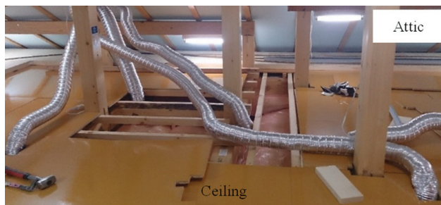
Fig. 2. Appearance of ducts installed in an attic.
