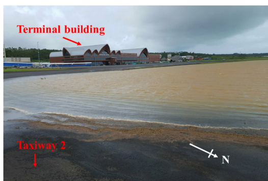
Fig. 4. Picture of the target site after the heavy rainfall event in February 2018.
