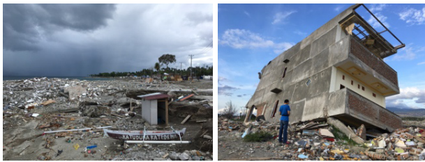
Fig. 3. The remains of a building after the liquefaction by a big Earthquake that hit Palu.
