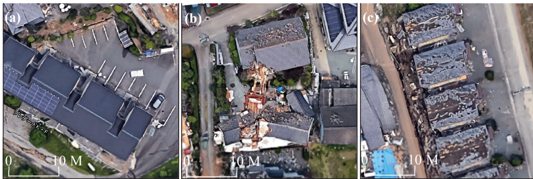
Fig. 6. Three examples of building damage patterns that caused misclassification: (a) oblique building; (b) vertical sinking building; and (c) building with tile damage.
