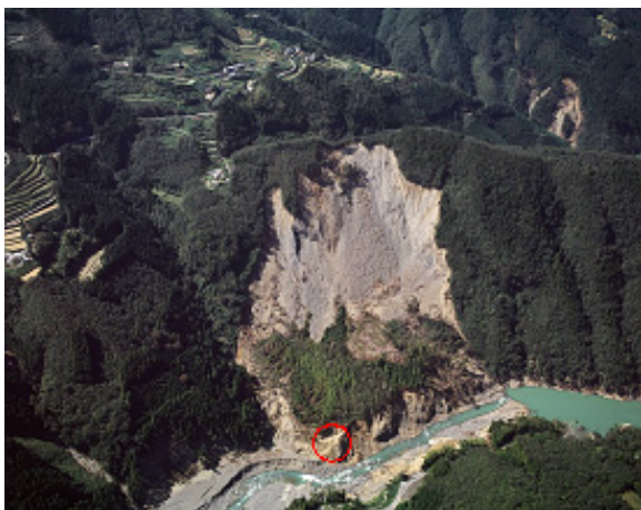
Fig. 2. Nonoo landslide dam after collapse.
