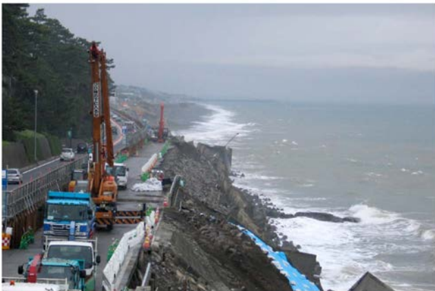
Fig. 7. Damaged Seisho Bypass seen from the top of the Ginpa Bridge looking east, October 8, 2007.
