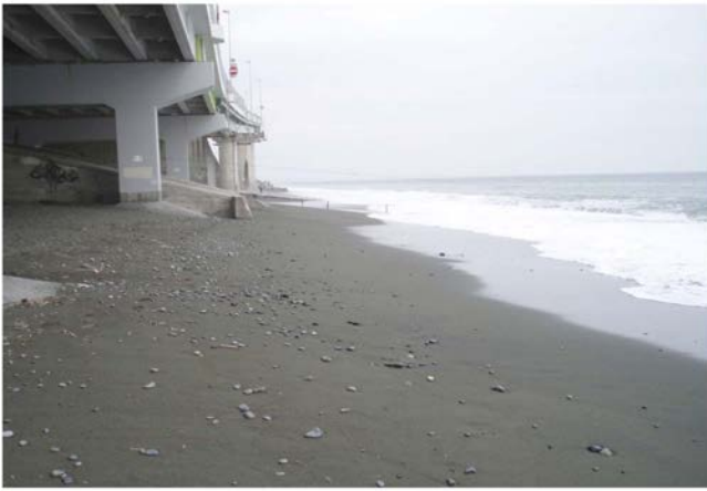
Fig. 14. 20-m-wide foreshore left under the Kinpa Bridge, September 4, 2007.
