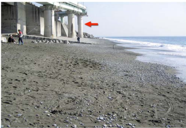
Fig. 15. Beach under the Ginpa Bridge, December 1, 2006.
