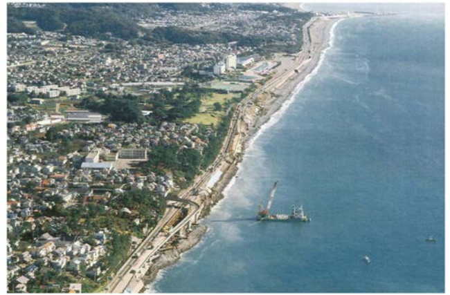
Fig. 9. Oblique aerial photograph of the damaged highway, November 13, 2007.
