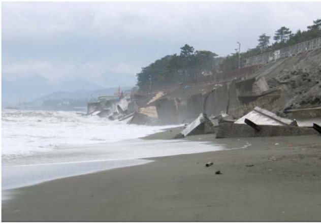
Fig. 6. Damaged highway and adjacent beach, October 8, 2007.
