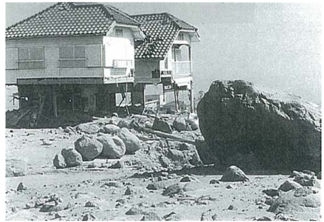
Fig. 5. A house damaged by debris flow.
