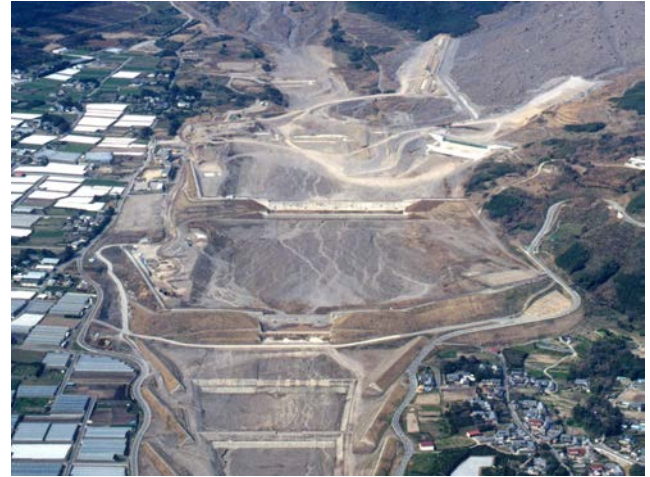
Fig. 10. Sabo dams and dikes were executed.
