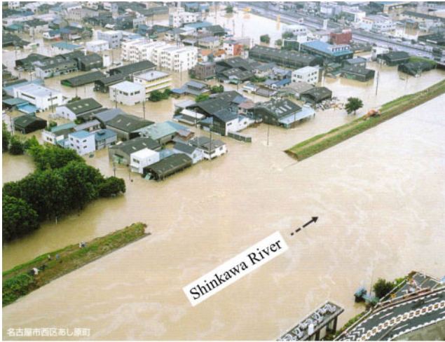
Fig. 5. Levee breach in the Shikawa River [2].
