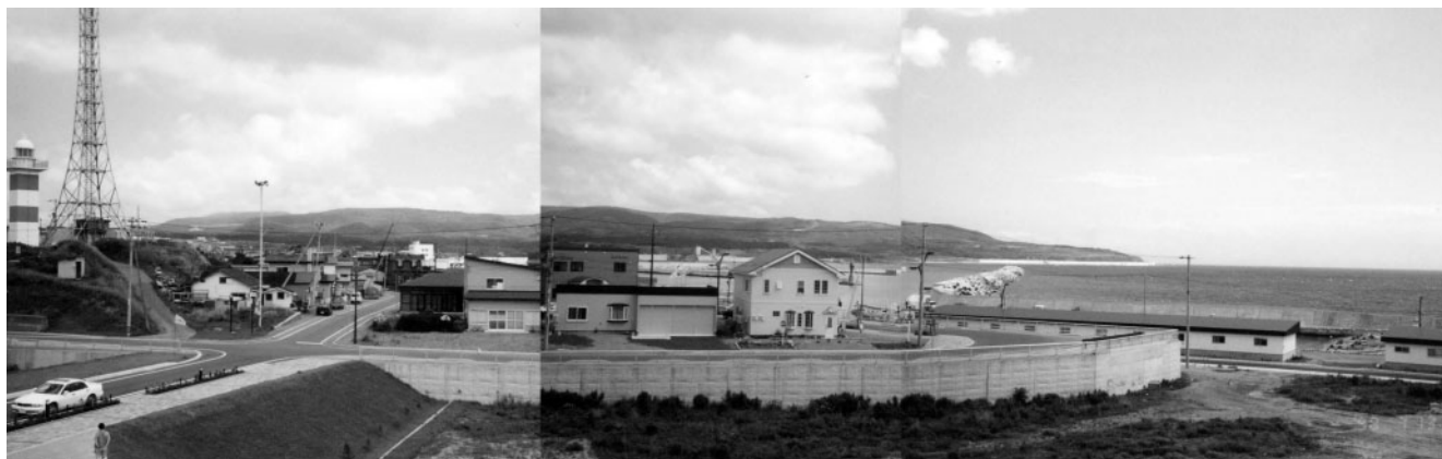
Fig. 6. Aonae division rebuilt by ground fill.
