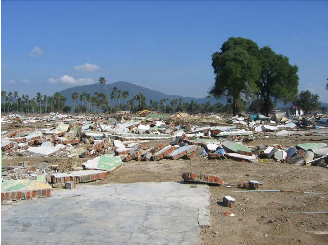
Fig. 4. Lhoknga Village on the west coast about 7 km southwest of central Banda Aceh. Only one house remained, that of Mr. Julpikar, near the right here.
